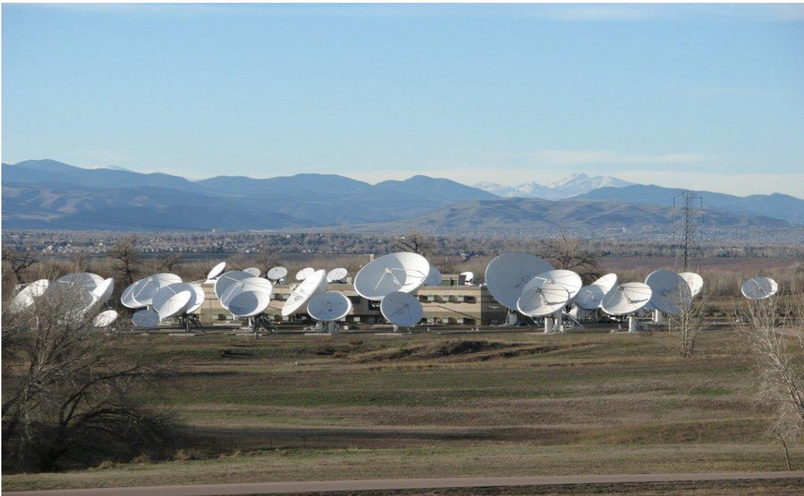
Figure 2: Typical Broadcast Antenna Farm of high gain satellite broadcast transmitters and receivers
